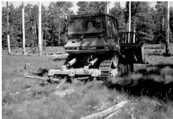
Figure 2. Severing lateral aspen roots using a tractor-mounted ripper. Coconino, NF, Arizona.
